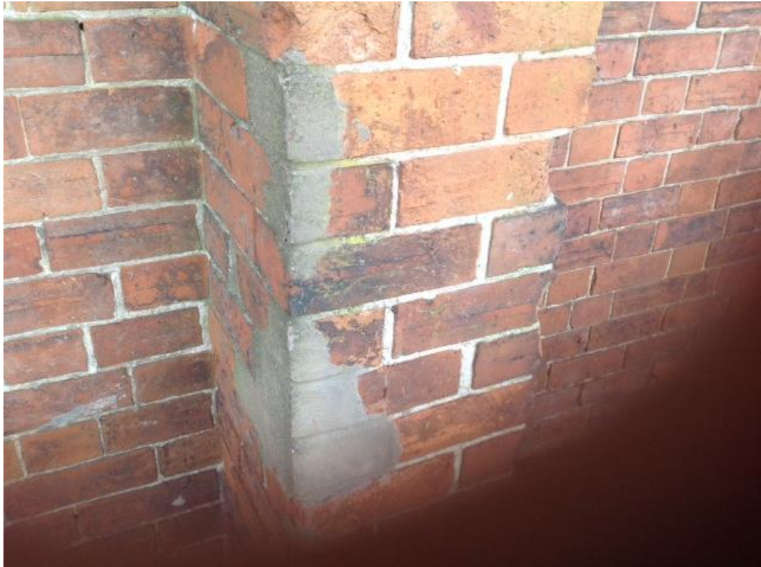
Image 12: Brick work pillar.
